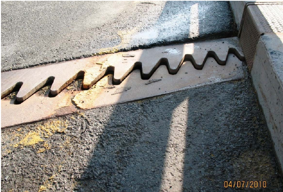
Vertically Misaligned Finger Joint (Bridge 17N shown)
