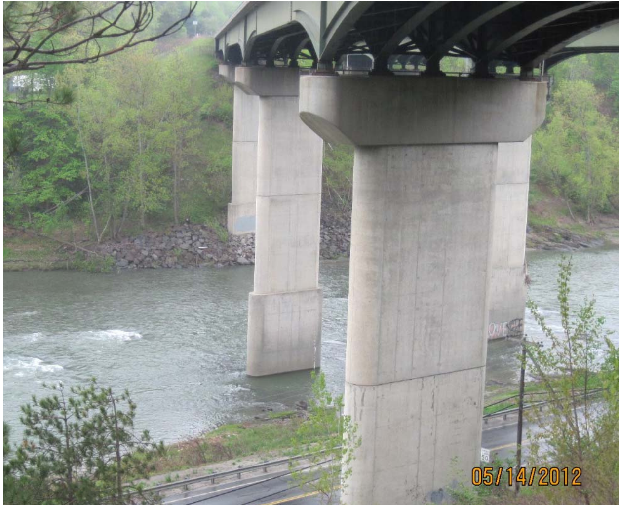
From embankment in front of Abutment #1 looking toward Pier #1, #3, and #5 (Below Bridge 17S)
