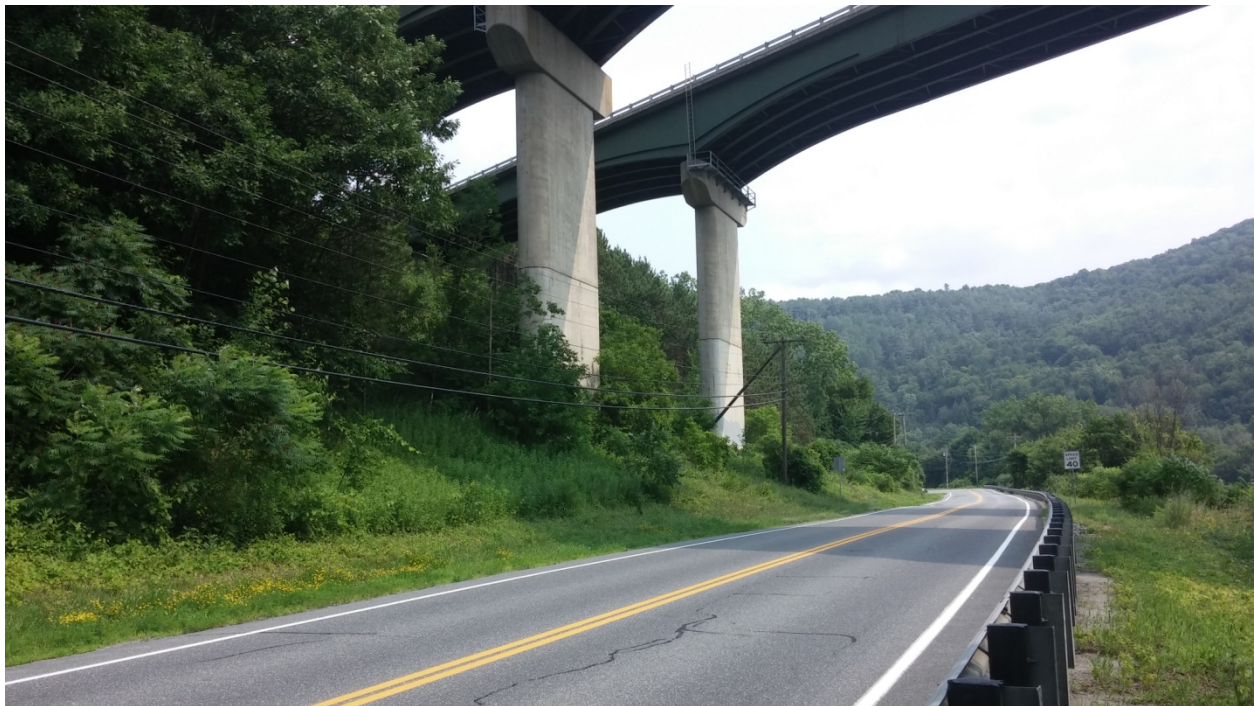
Figure 2: Bridge Piers Looking East
