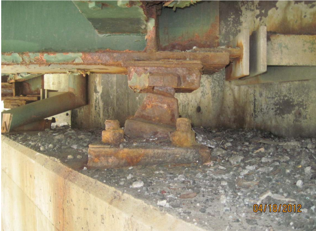
Tilted Bearing (Bridge 17N shown)
