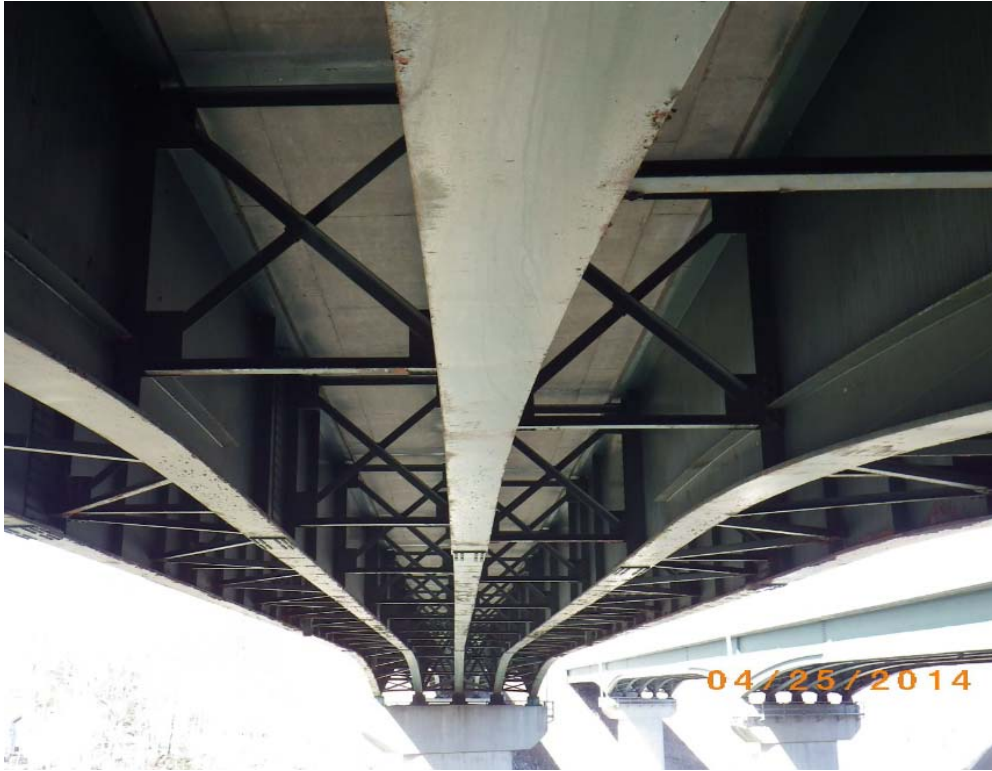
Underside of Bridge (Bridge 17S shown)
