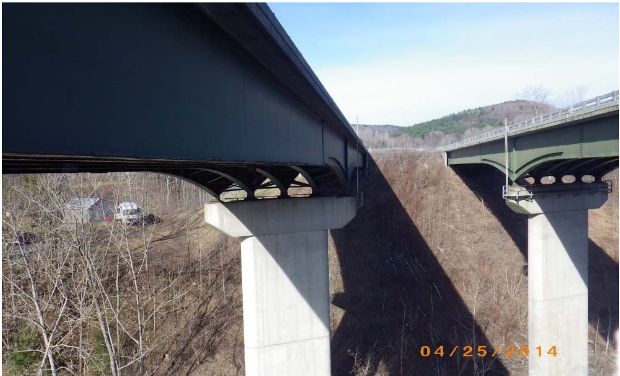
From Span 3, Bridge 17S - facing Abutments 3 and 4
