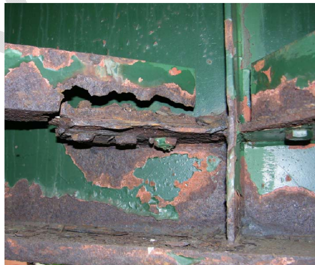
Figure 2: Lateral Bracing Deterioration below Drip Tubes
