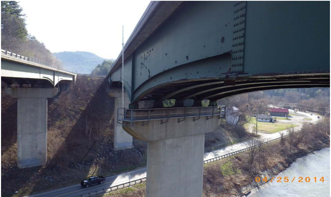
From Span 3, Bridge 17S (VT Route 14 below)
