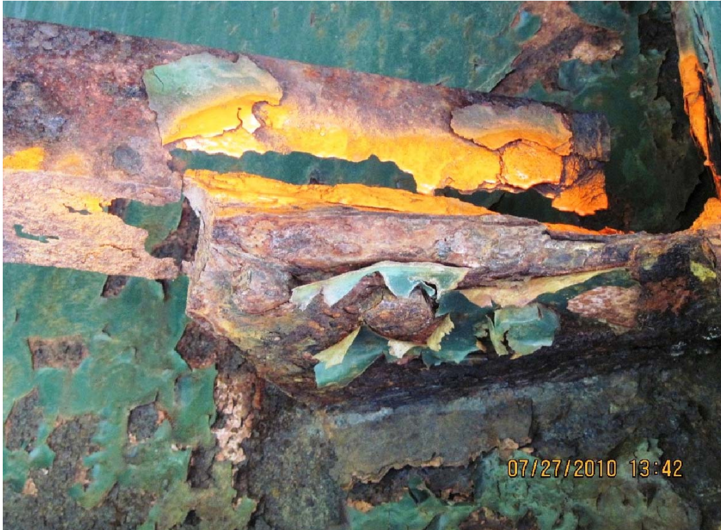
Lateral Bracing Angle Deterioration below Deck Drip Tube (Bridge 17N shown)
