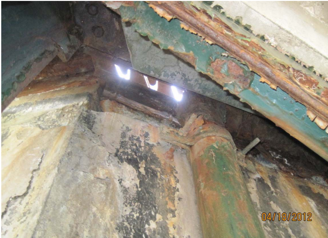
Exposed Finger Joint (Bridge 17N shown)
