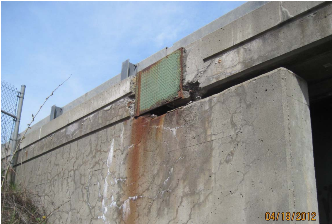
Wingwall and End of Deck (Bridge 17N shown)
