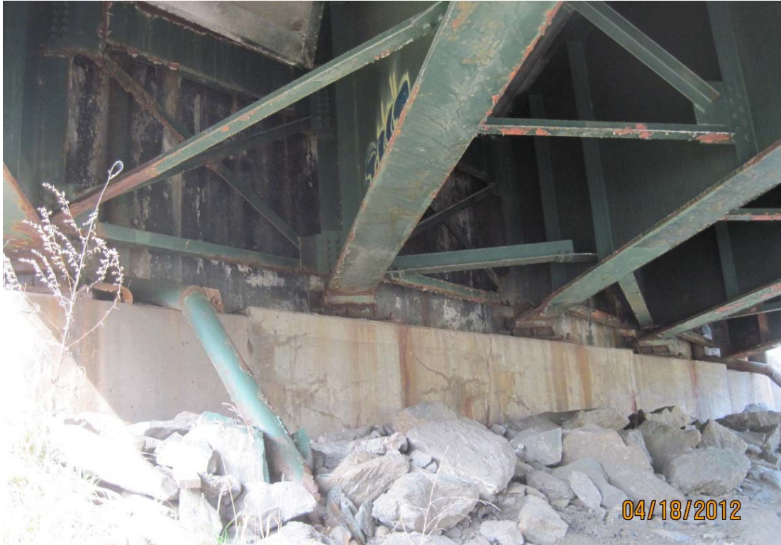
Condition of Abutment and Backwall (Bridge 17N shown)
